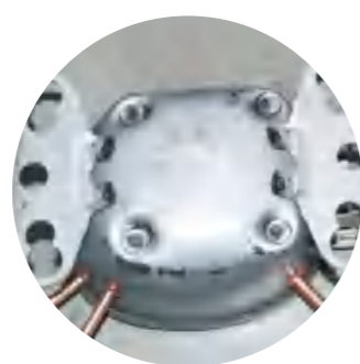
机脚焊接 Welding Of Base Legs
